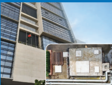
Restricted Facilities Building Project Name: Bangladesh Secretariat Capacity: 500 m 3 /day
