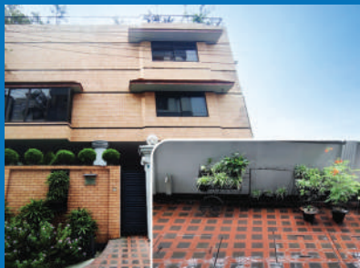
Existing Building Project Name: Saif Mansion (ABC House) Capacity: 5 m 3 /day
