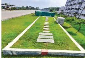
Project Name: 66 Bengal Capacity: 100 m 3 /day
