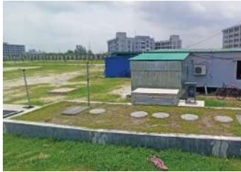
Project Name: 12 Signal Capacity: 40 m 3 /day
