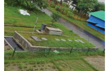
Project Name: DIV. Headquarter Capacity: 40 m 3 /day
