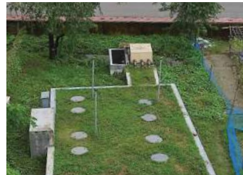
Project Name: MES Barrack Capacity: 40 m 3 /day
